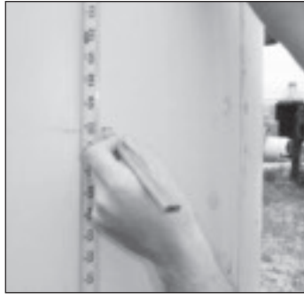
1. Measure and mark finished porch height.
