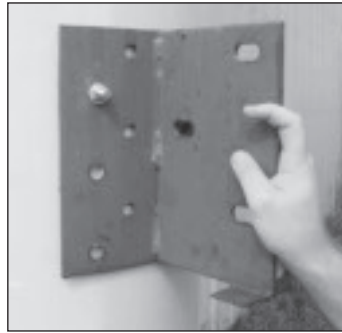
5. Apply bracket support tab and hand tighten bolt.
