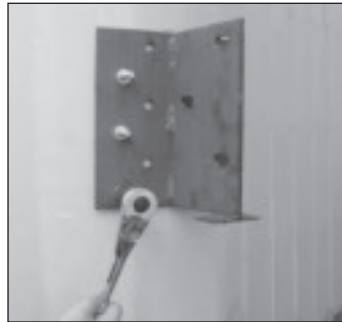
7. Drill remaining holes and tap in remaining anchors and secure. (Refer to note 4 and tips.)
