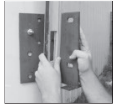
6. Level bracket and drill remaining 5 holes.
